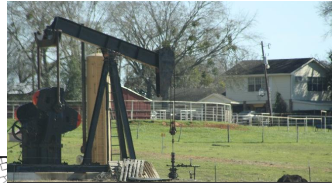
Existing vertical oil production
