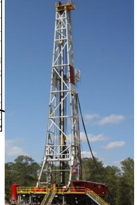
Rig drilling 6,000 ft lateral in Woodbine
